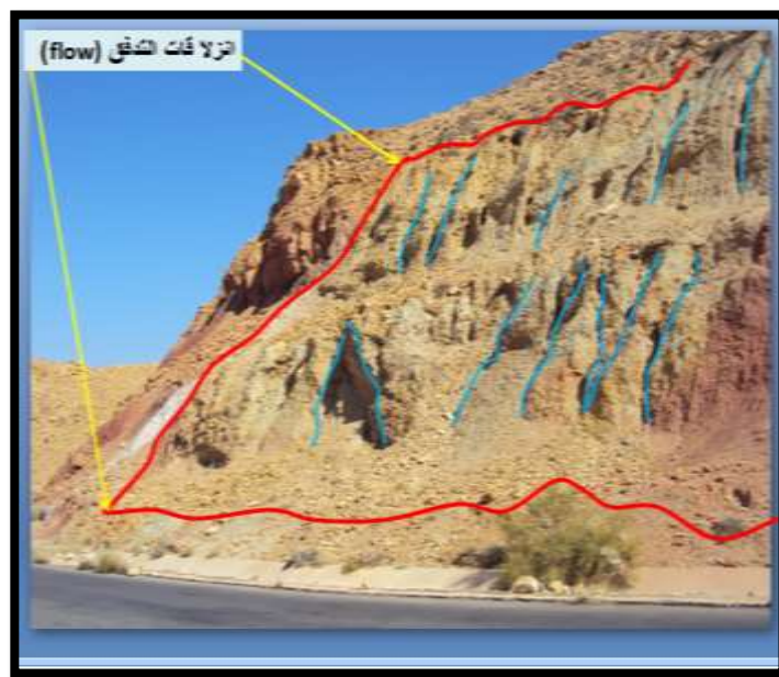
Figure (9): Shows the flow-type landslides present at the second site in the Al-Hamra area, which occur as a result of the mixing of particles accompanied by movement.
