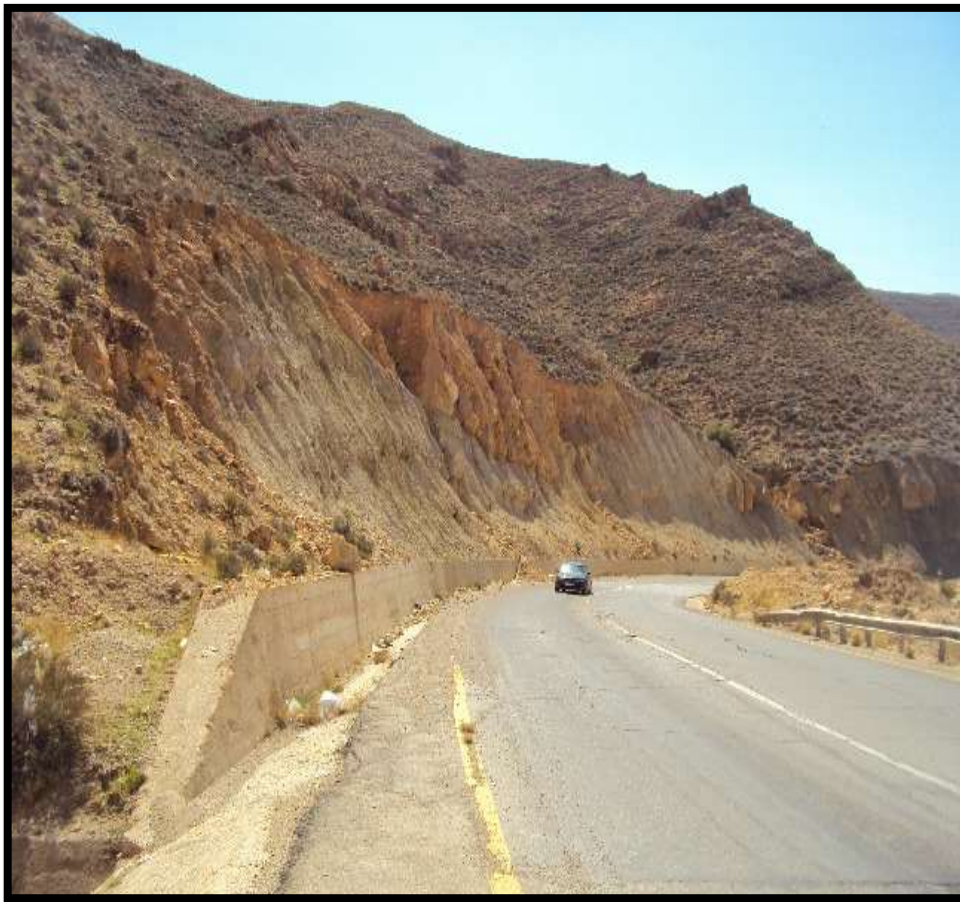
Figure (10): Shows the flow-type landslides present at the second site in the Al-Hamra area, which occur as a result of the mixing of particles accompanied by movement.
